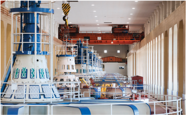
Hydro Electric Power Turbine Generators
